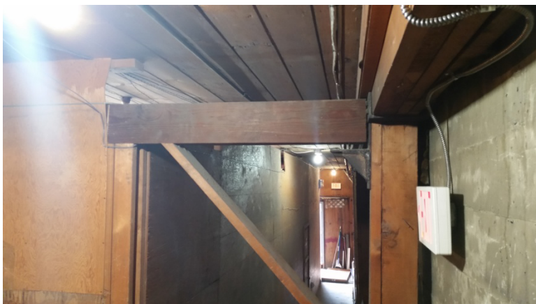
Figure 4 Gap at settled column
