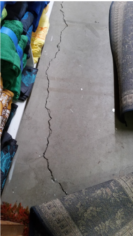
Figure 10 Crack in slab in storeroom
