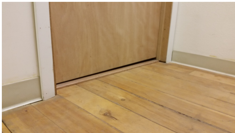
Figure 7 Slope in floor at door sill
