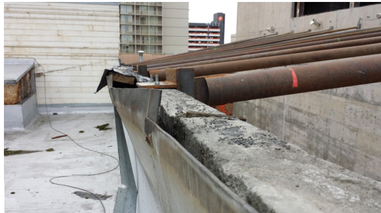
Figure 12 Open top of common wall
