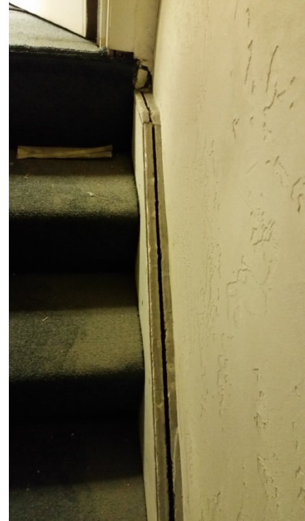
Figure 3 Separation at west side of stair
