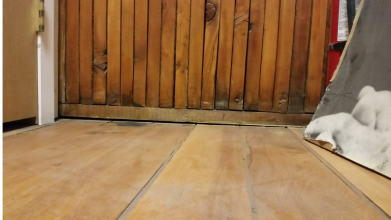
Figure 8 Slope of floor at interior wall
