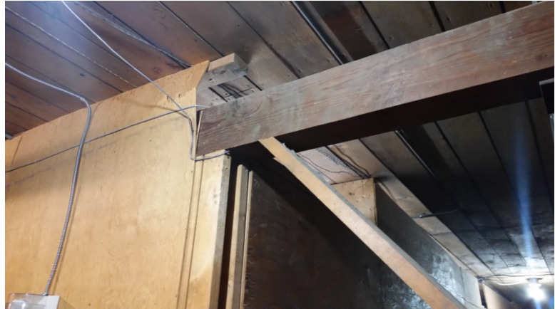
Figure 5 Buckled plywood
