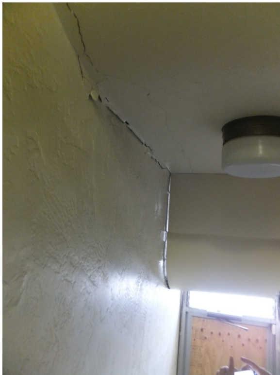
Figure 1 Separation at west wall of stair
