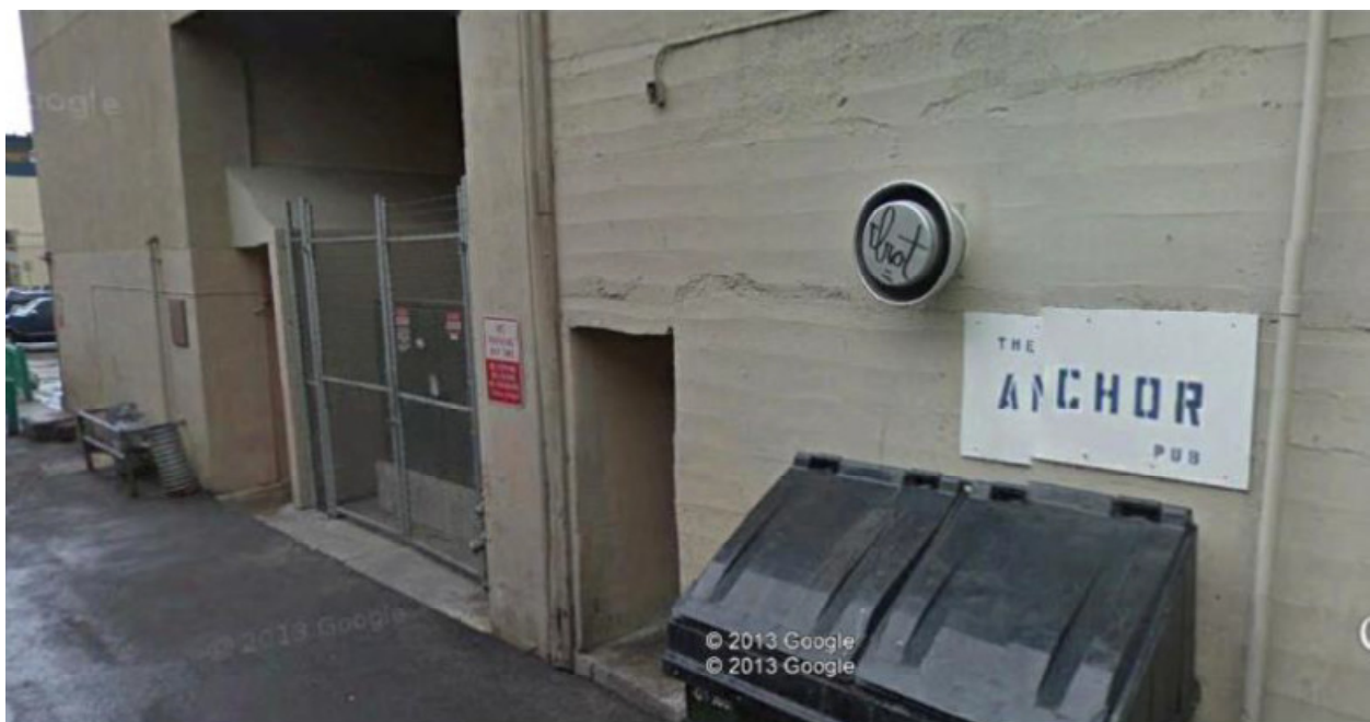
Photo 29: South Wall of Anchor Pub
