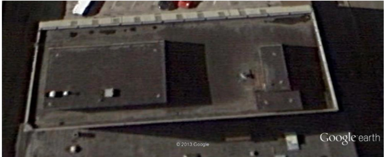
Photo 5: Ariel View #5 LIO Roof
