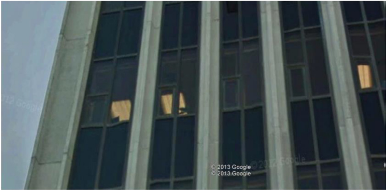
Photo 7: North Elevation Close Up
