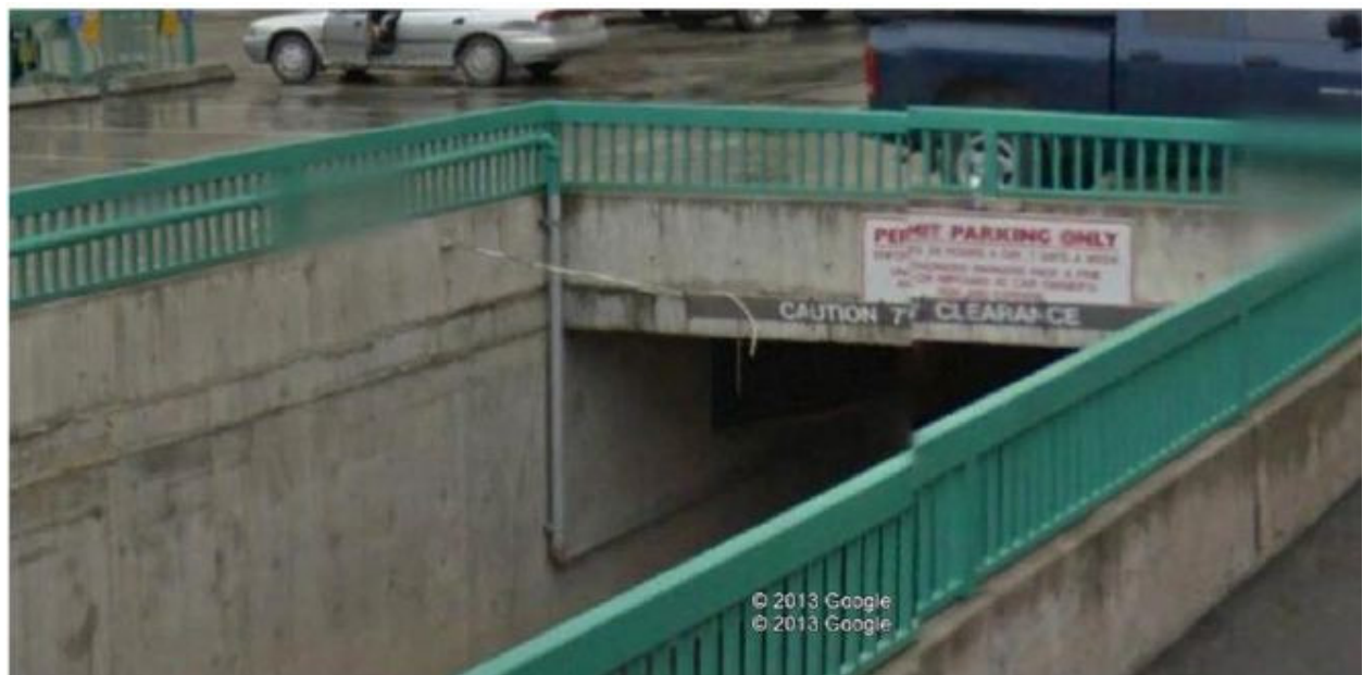
Photo 21: Parking Garage Close up
