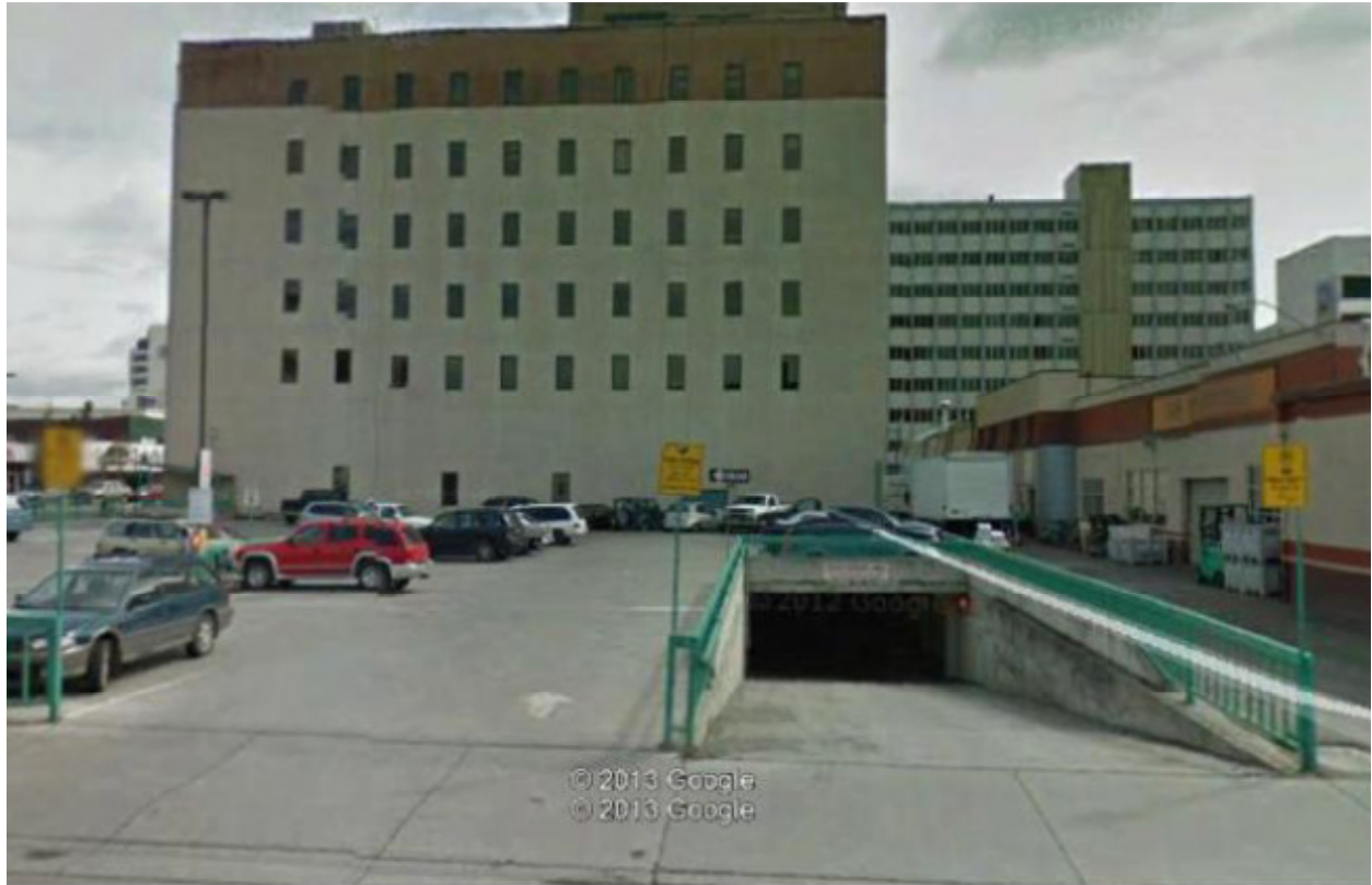
Photo 18: Parking Ramp and West Elevation
