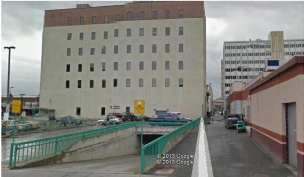
Photo 20: Parking Ramp and Alley
